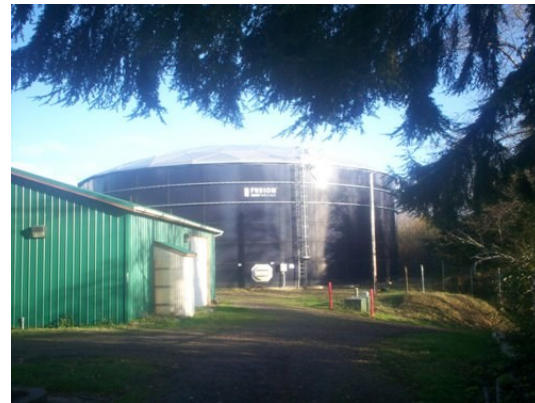
City of Nehalem Water Treatment Plant & Reservoir
