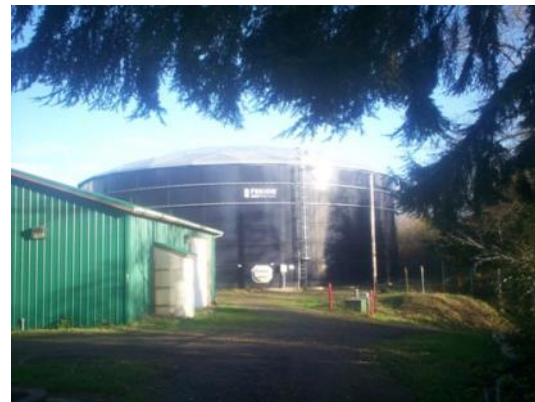
City of Nehalem Water Treatment Plant & Reservoir
