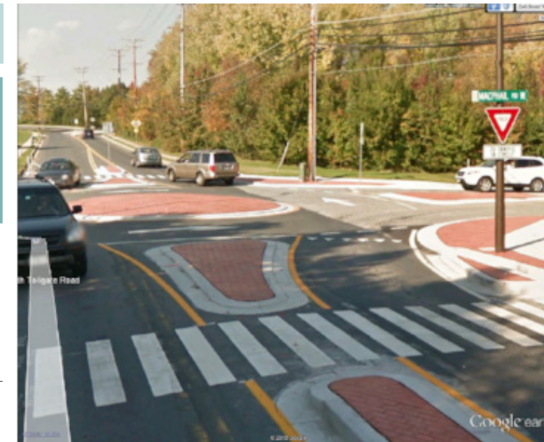
Example of a mini-roundabout with a traversable center island designed for trucks to drive over. Photo Source: Transportation Research Board
