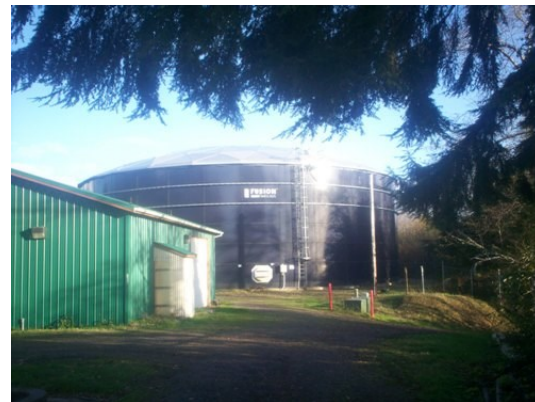
City of Nehalem Water Treatment Plant & Reservoir
